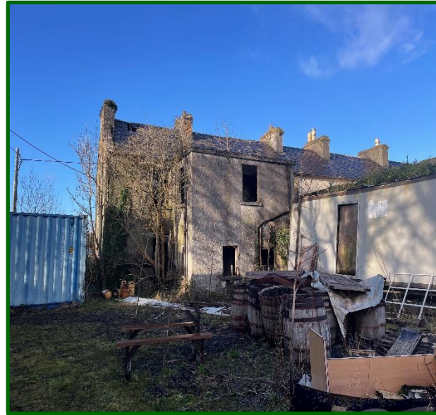
Picture 2: Buildings and Artificial Surfaces (BL3) on-site
